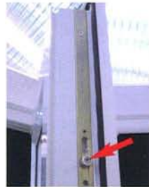
Oil door locking pins and shoot bolts
