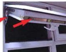
Oil friction stays (hinges) and window locking pins Oil door locks and latches
